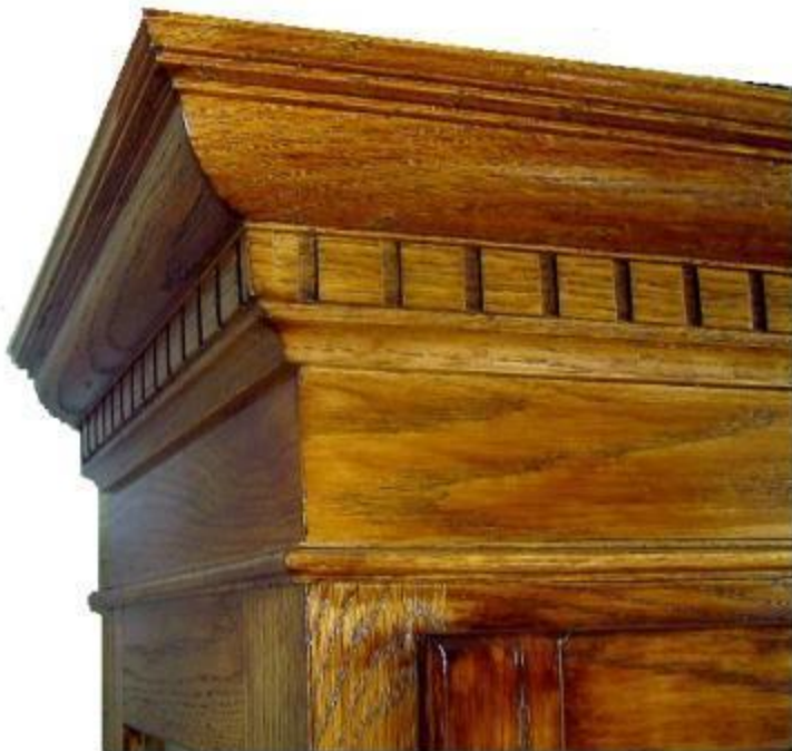
Dentil Moulding
